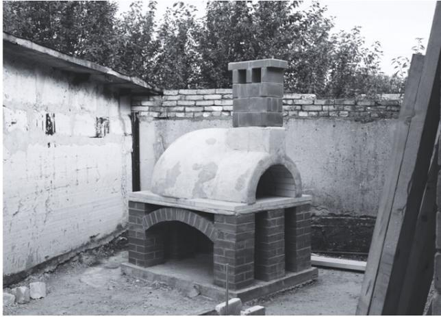
The stove itself is a small brick igloo with a pipe, and sits on a cement table, which makes it easier to use, helps retain heat, and protects against possible fires. The pipe is covered with cement mortar. Under the "dome" of the furnace itself, there is an empty space for the firewood, closed by a steel door. The door was cut and soldered according to Enrique's design at a local laser-cut metal shop, with the help of one of Kulgu residents.
